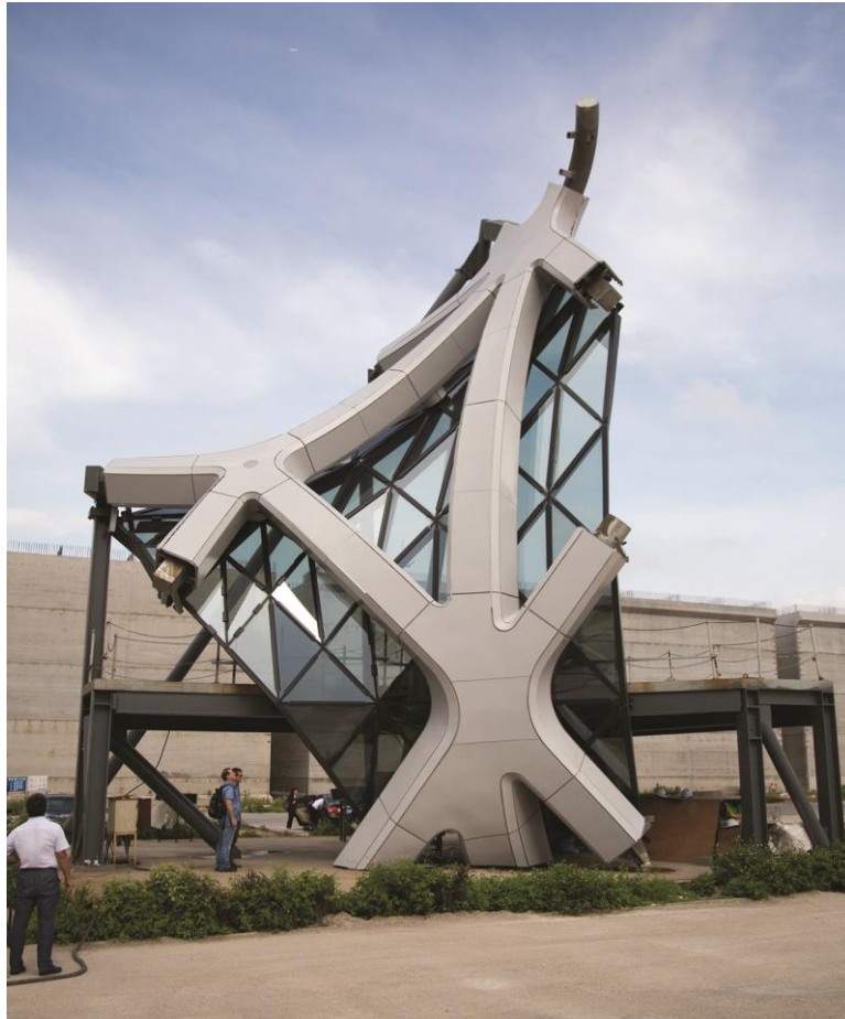
Figure 26. Completed visual mockup for City of Dreams (used courtesy of the authors with permission)
